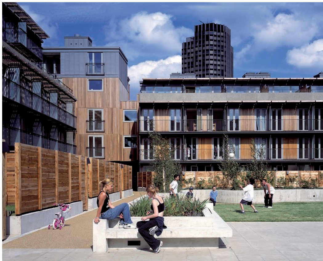
Iroko Housing Co-operative, logement social à Coin Street, Arch. Haworth Tompkins Limited © Morley von Sternberg
