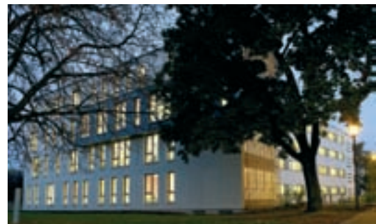
Manufacture, Atelier d'architecture Simon Teyssou, © architectes
